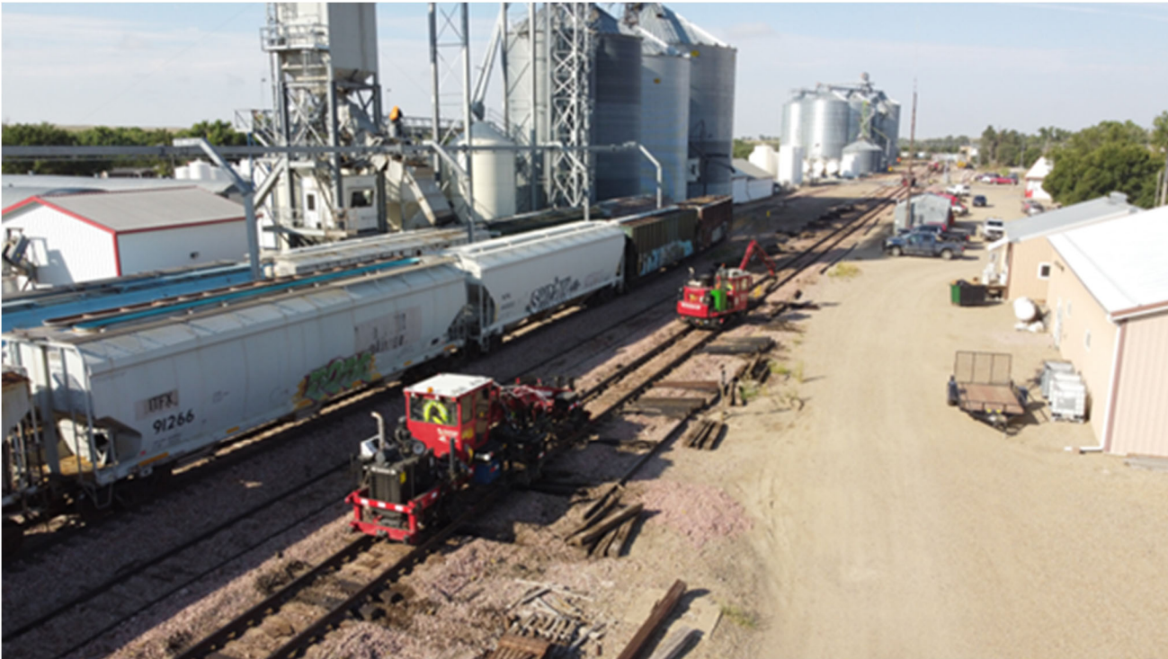
8/28/25 Tie replacement in Phillip
