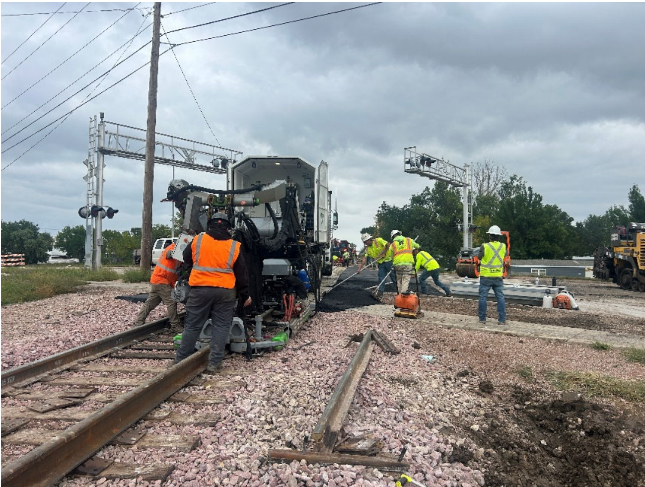
9-17-25 Asphalt paving and rail relay through Lacrosse Street in Rapid City
