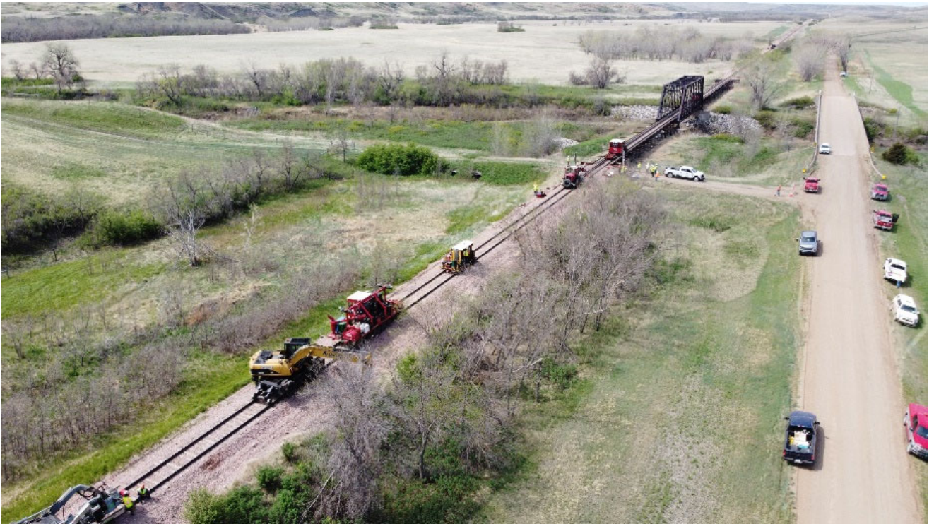
7-25-25 rail relay crew near MP 496.5
