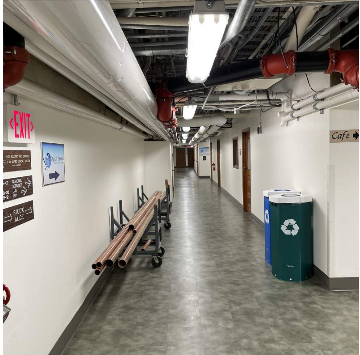
▲ Basement Level: Corridor viewing west
