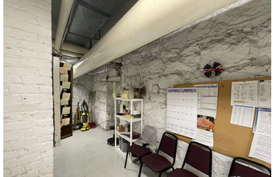
▲ Basement Level: Custodial space
