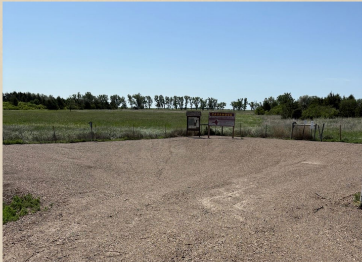
Casanova GPA Parking Lot Improvement
