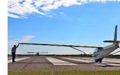
View of Watertown Municipal Airport Runway
