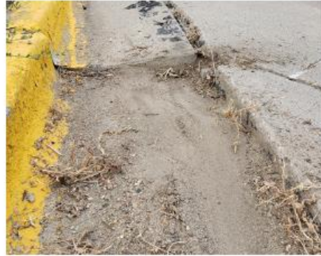
Settled curb in employee parking lot
