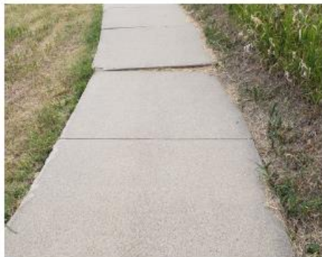
Southwest corner of visitor parking lot
