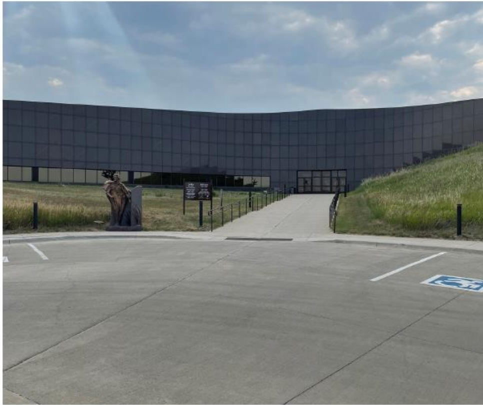
Front of building windows
