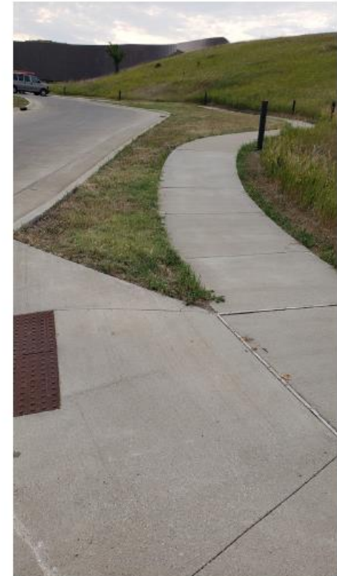
Southwest entrance of visitor parking lot
