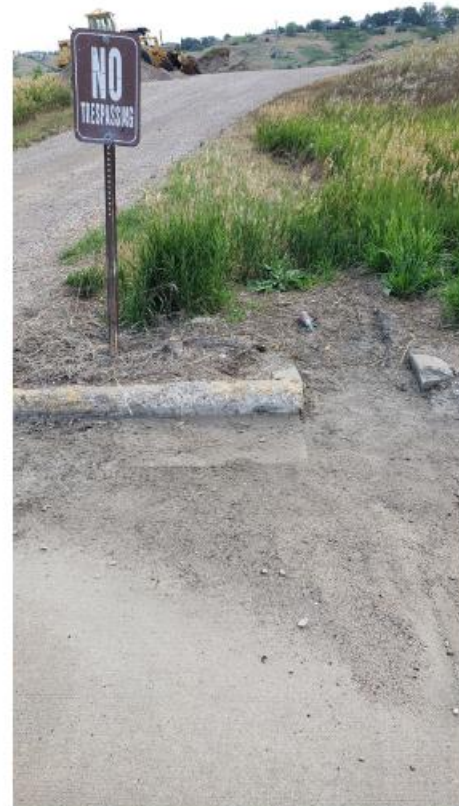
Sediment build-up in employee parking lot
