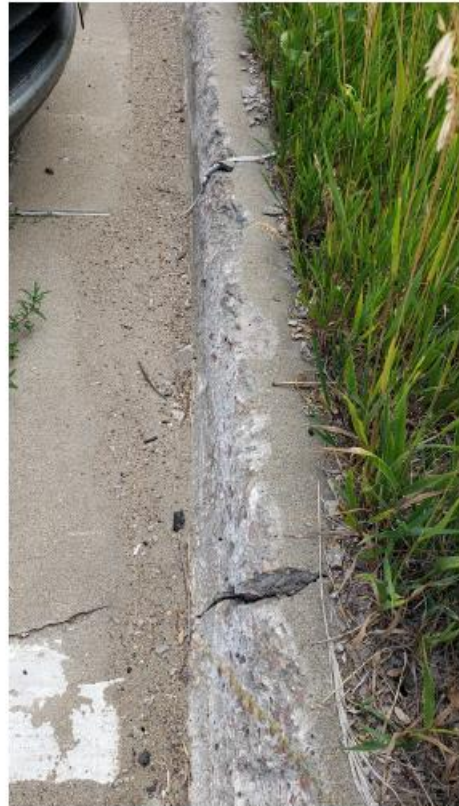
Chipped curb in employee parking lot
