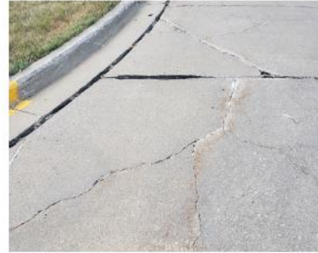
Cracked pavement in employee parking lot
