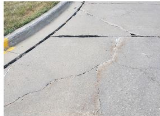
Cracked pavement in employee parking lot
