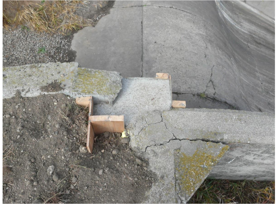
Repair completed with rebar and concrete to prevent wing wall collapse
